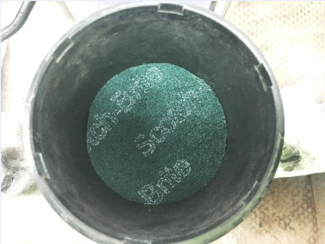
New Scotch Brite Screen in place
