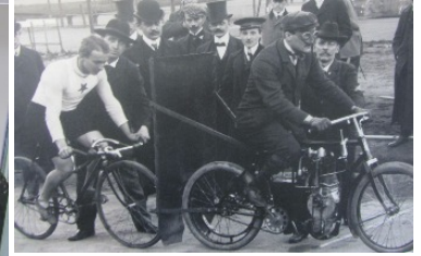
1910 Kolem windbraker for bicycle record attempt, it has no gearbox.
